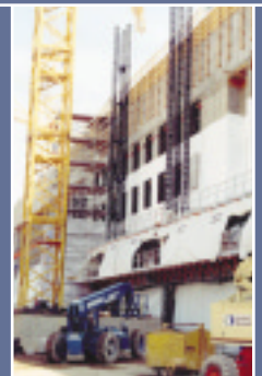
Combined features! The Pentagon Reconstruction Project shows superimposed decking with weather enclosure, 910 kg (2,000 lbs.) monorail in the front and a special triple mast base allowing freestanding work to a height of 24 m (78 ft)!
